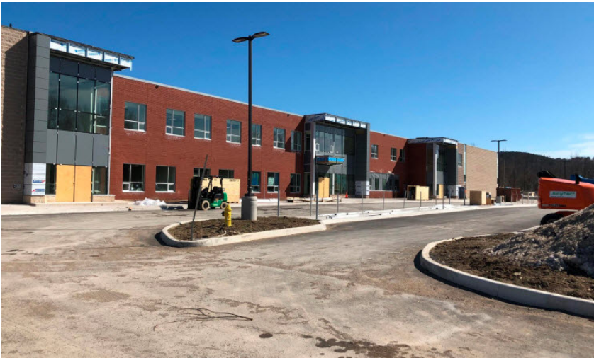
Georgian Bay Community School build project
